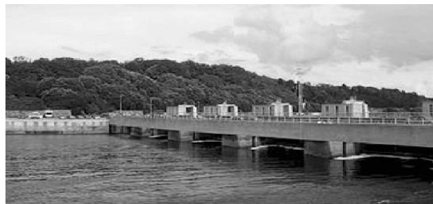
Fig. 5. The world's first tidal power plant, La Rance, France [5]
